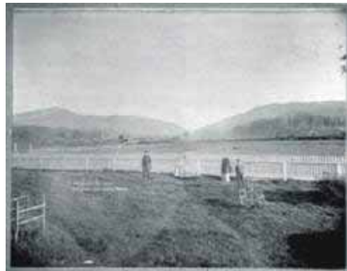
Anderson Farm looking south past Pickering Barn
